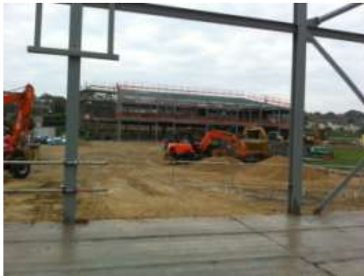
Figure 9.4 'From unearthing values to building foundations' - TSS under construction September 2013
